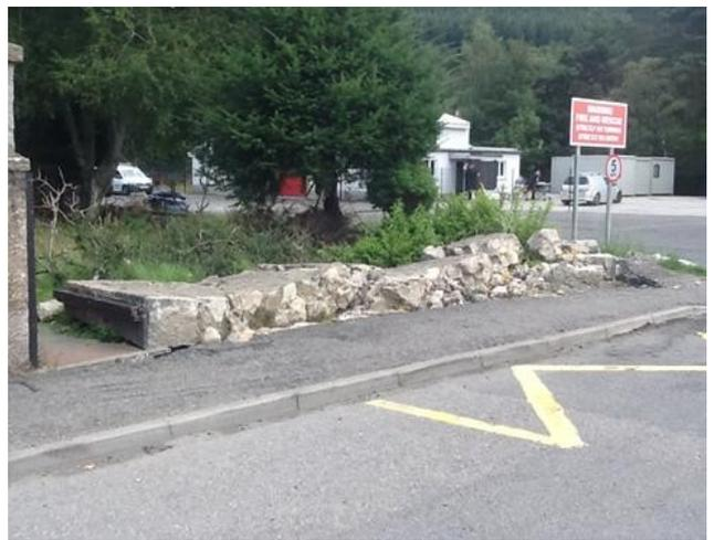
The wall at the fire station, which was brought down by the force of the water.
